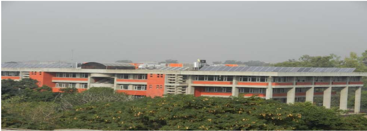
Rooftop SPV system (50 kWp) at ParyawaranBhawan, Chandigarh
