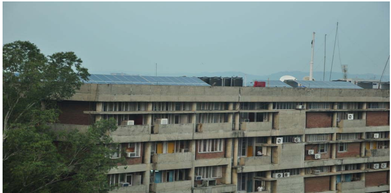
25 KWp SPV Plant at Police Hq, Chandigarh
